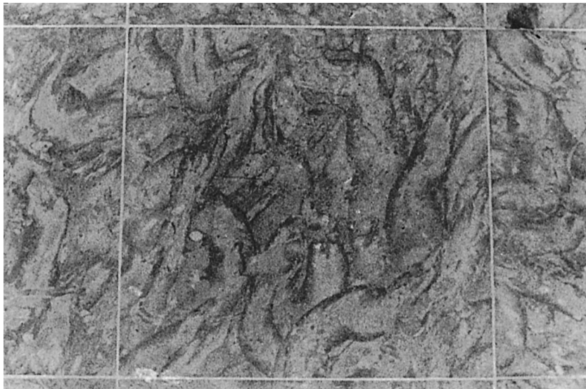
Fig. 3. Close-up of the cladding slabs of echinoid-burrowed sediment ( Bateig Fantasia ) on the upper floor of Fenwicks.
